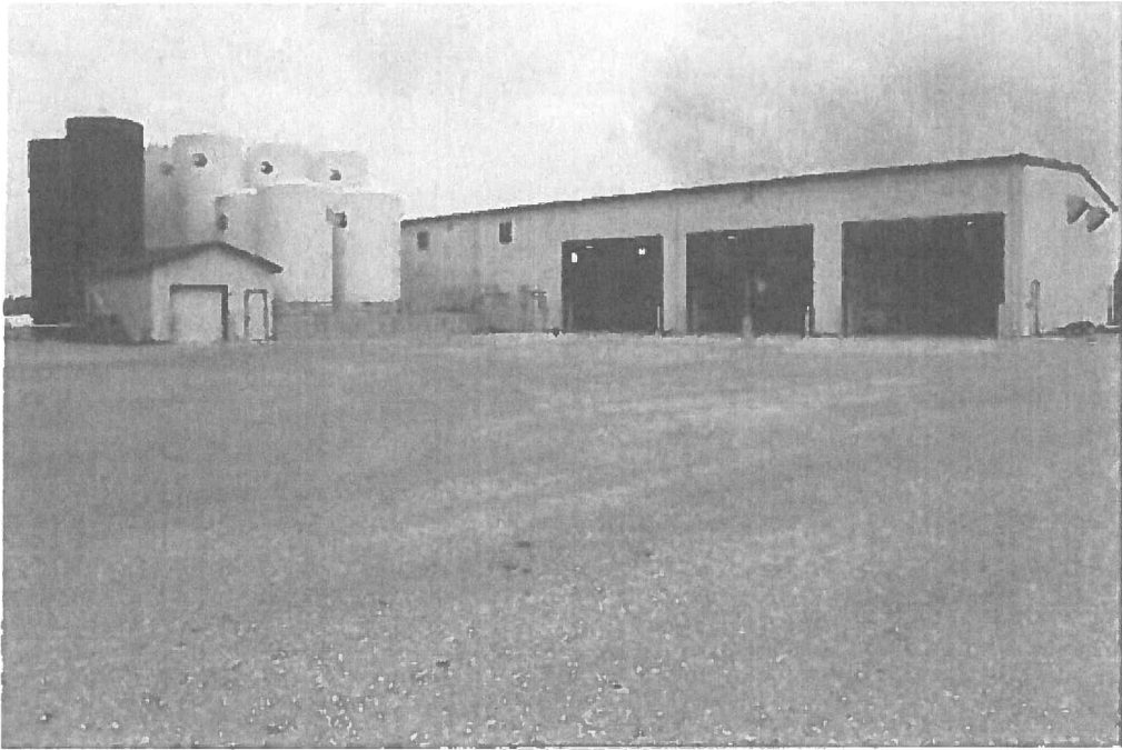
West Side of Liquid Fertilizer and Chemical Building
