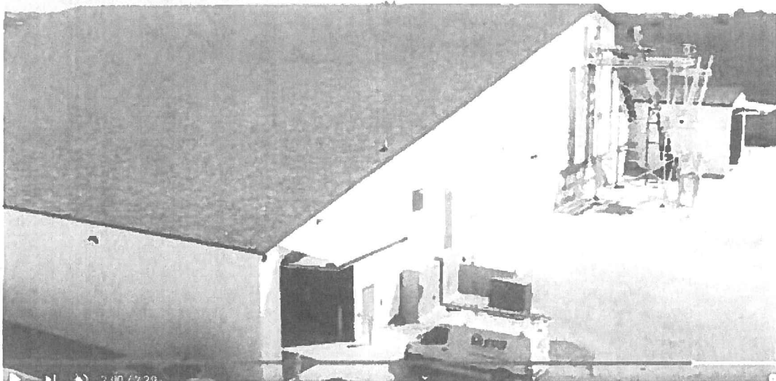
West and North Side of Dry Fertilizer Building
